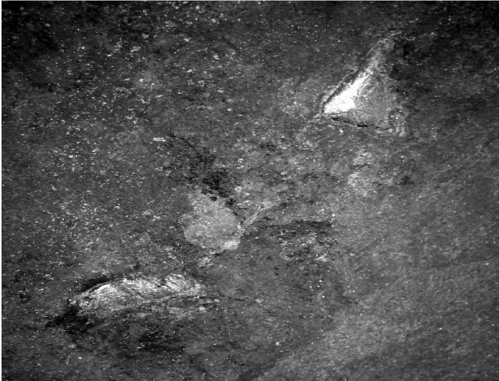
Figure 8. Internal defect on the heat exchanger cover
